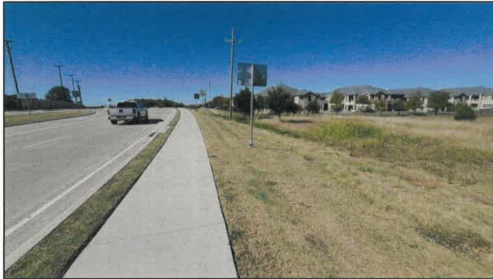
VIEW OF TEXAS 276 LOOKING WEST
