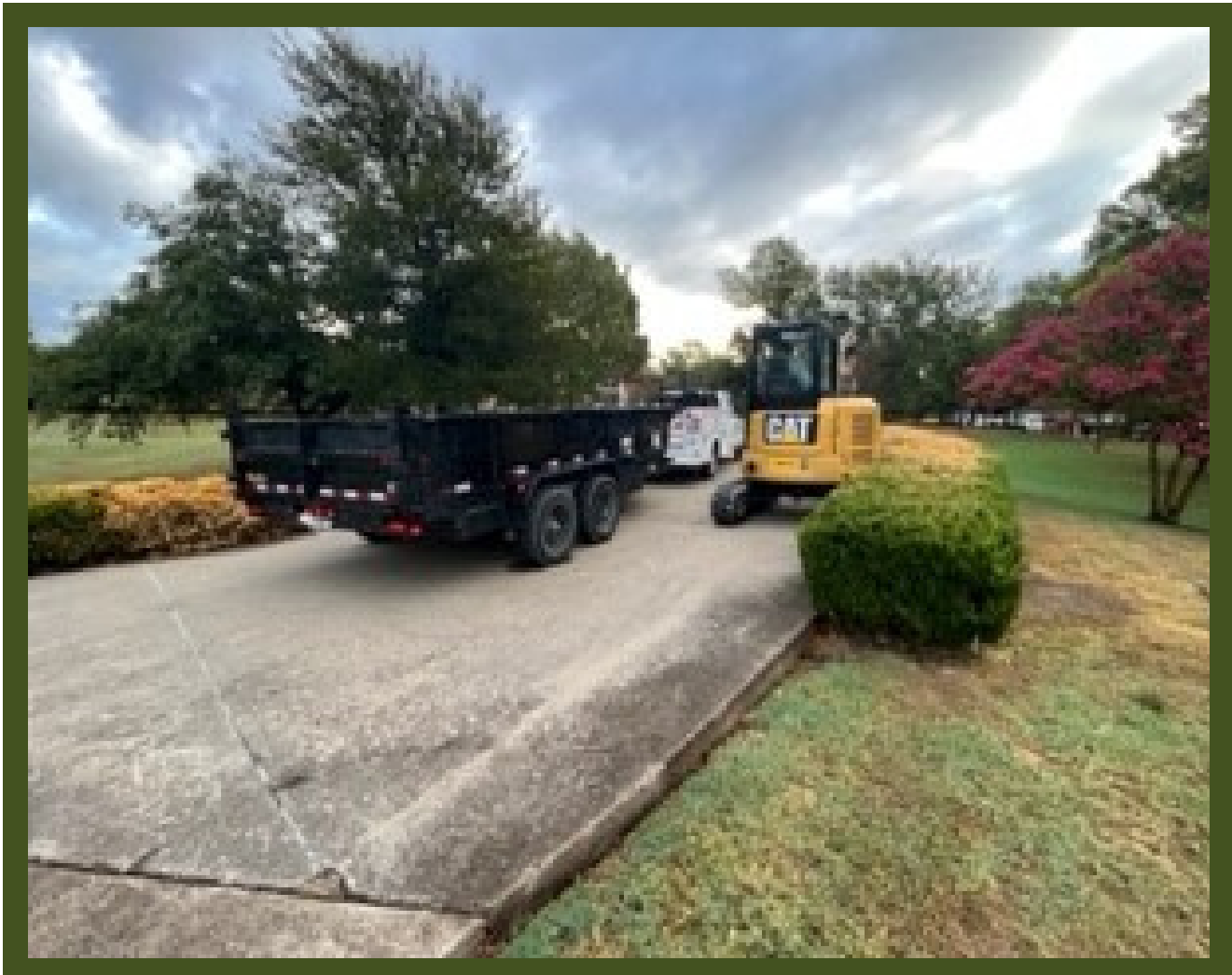
CITY HALL BOX WOODS REMOVAL
