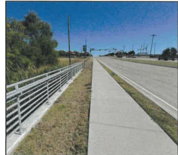
VIEW OF TEXAS 276 LOOKING EAST FROM THE CULVERT CROSSING TX 276
